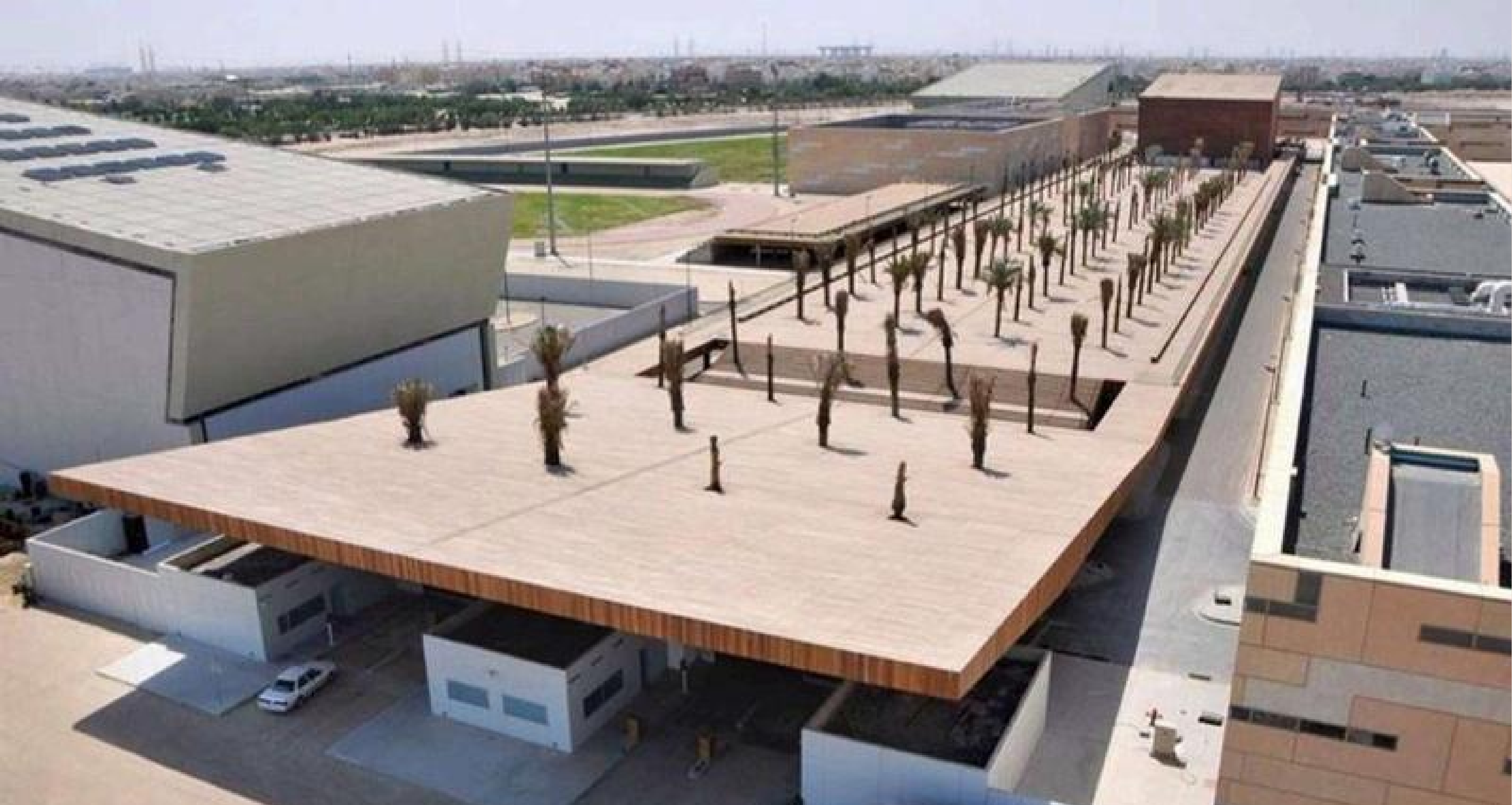
Kuwait Police Academy , SOM - 2012 , 50,000 m2 , 2000 tonnes of prefabricated IPE cladding panels to parade ground and 5 storey auditorium
