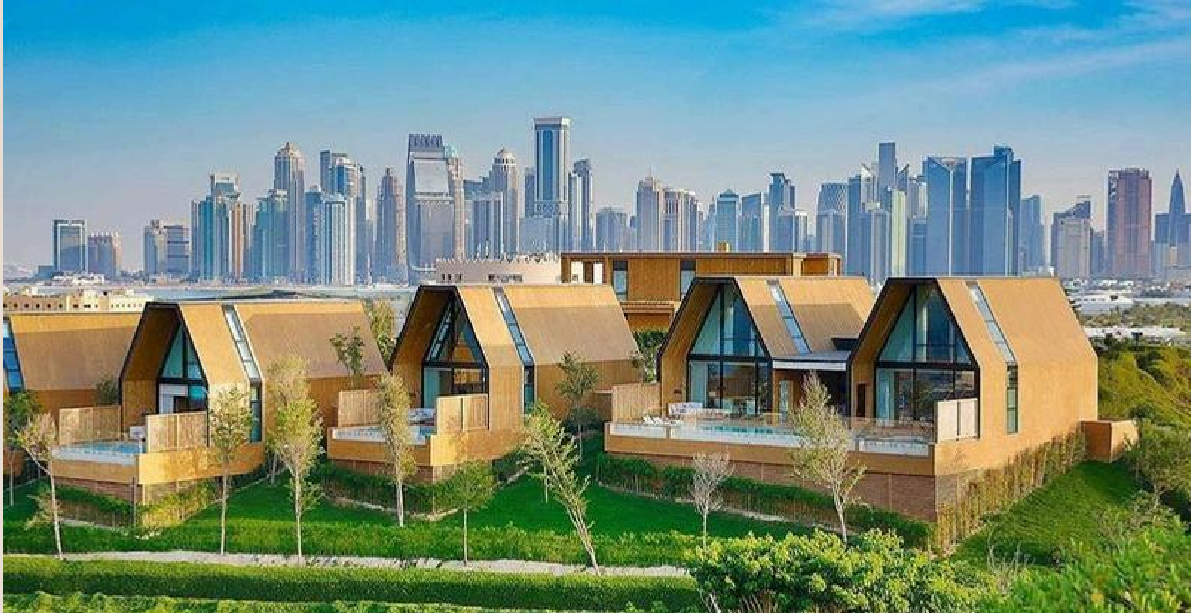
KATARA Hills, Qatar, 2022 ; Steel moment frames with Prefabricated Indian plantation hardwood LVL Panels cladded with Thermowood- Constructed 14 VIP Villas in time for the FIFA 2022 World Cup on a rushed 16 weeks schedule from award.
